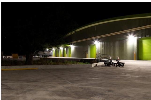
Downlighters tucked underneath an overhanging canopy close to the building light walkways whilst minimising spill into adjacent areas. This also helps to reduce the effect of night lighting when seen from above from high ground close by.
