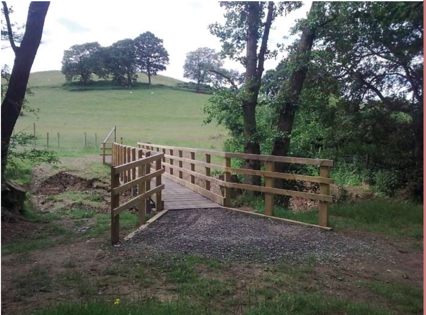
New footbridge, Storridge
