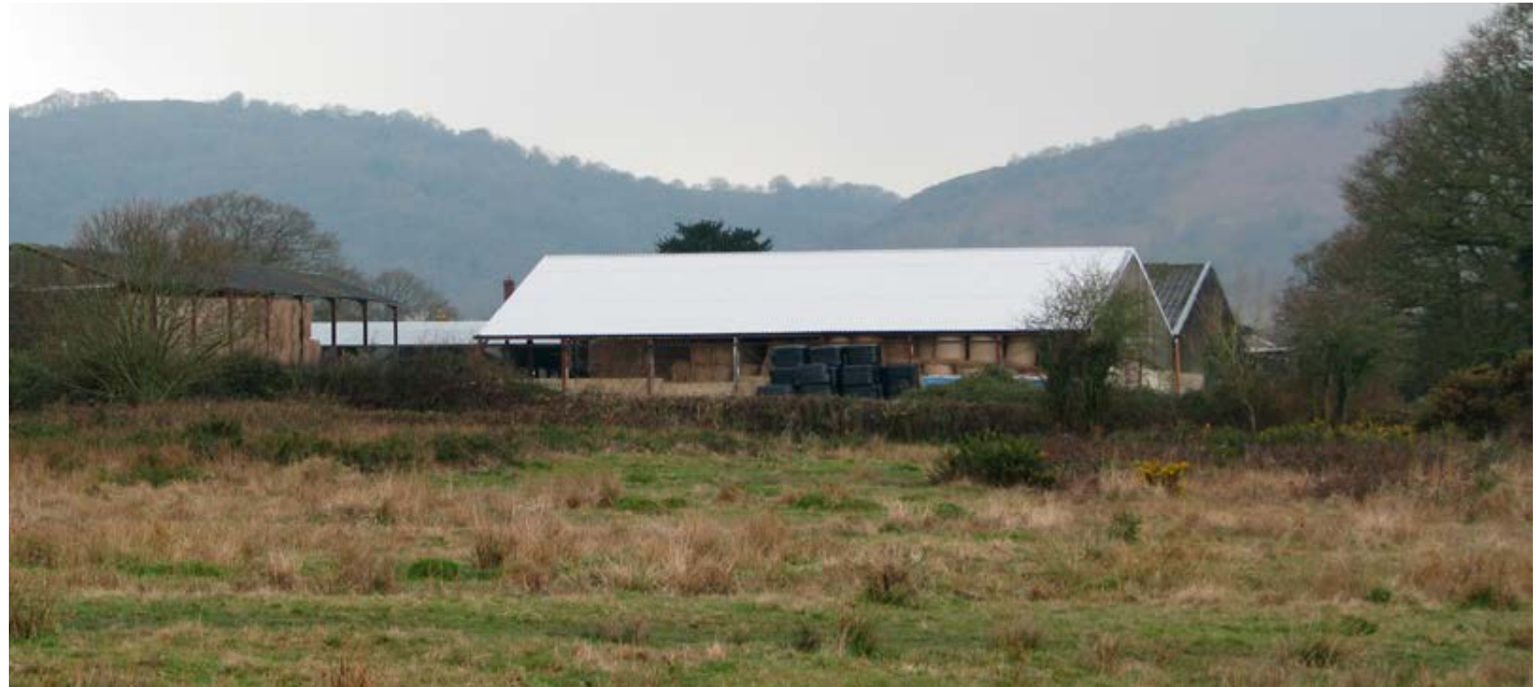
Highly reflective roofing material
