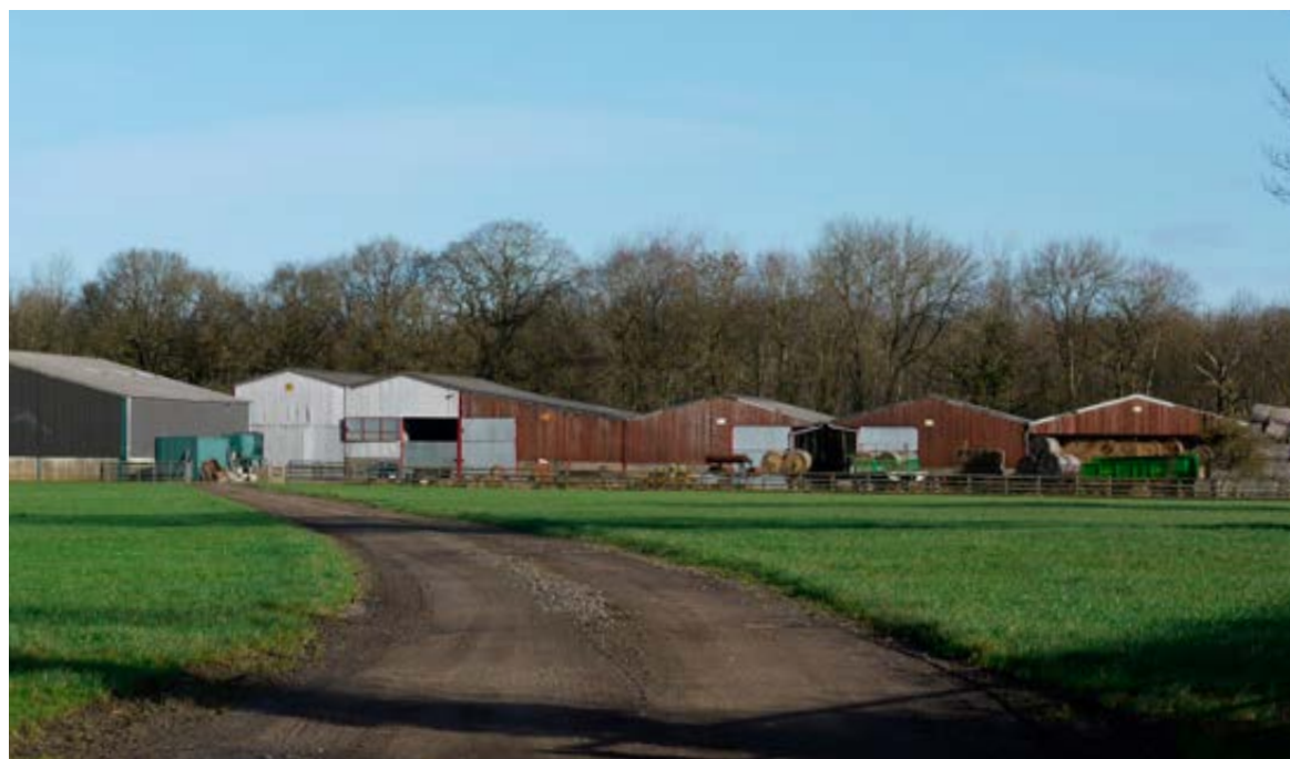
Partly right, partly wrong: light coloured doors and too many materials
